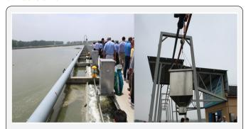
Figure 2: Air lift pump at the inlet point and automatic feeders.
